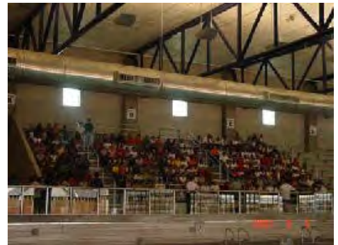
Stadium seating view
